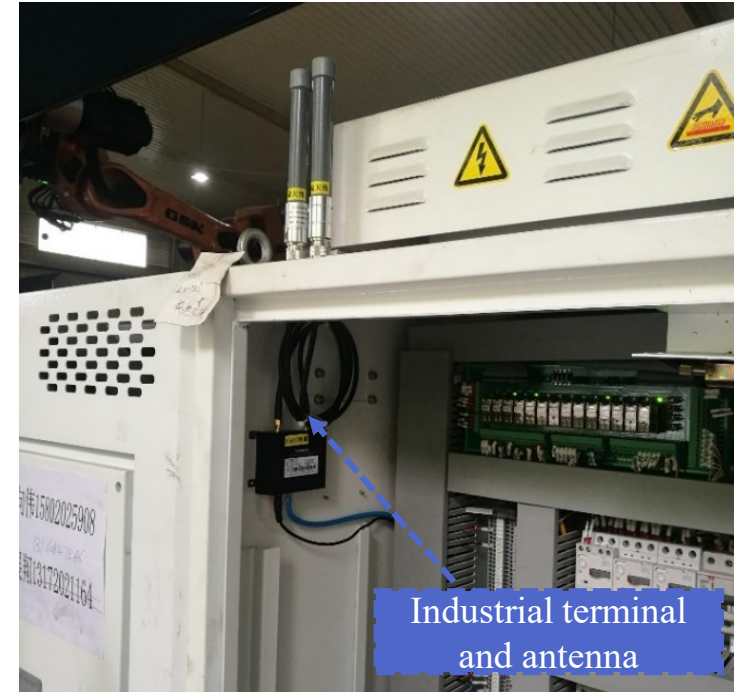
Industrial center access equipment and antenna
